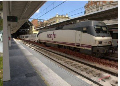
Valencia Train Station, Spain
